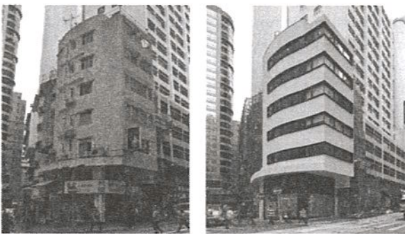
Before and After the renovation of the building, in which the apartments were built in
